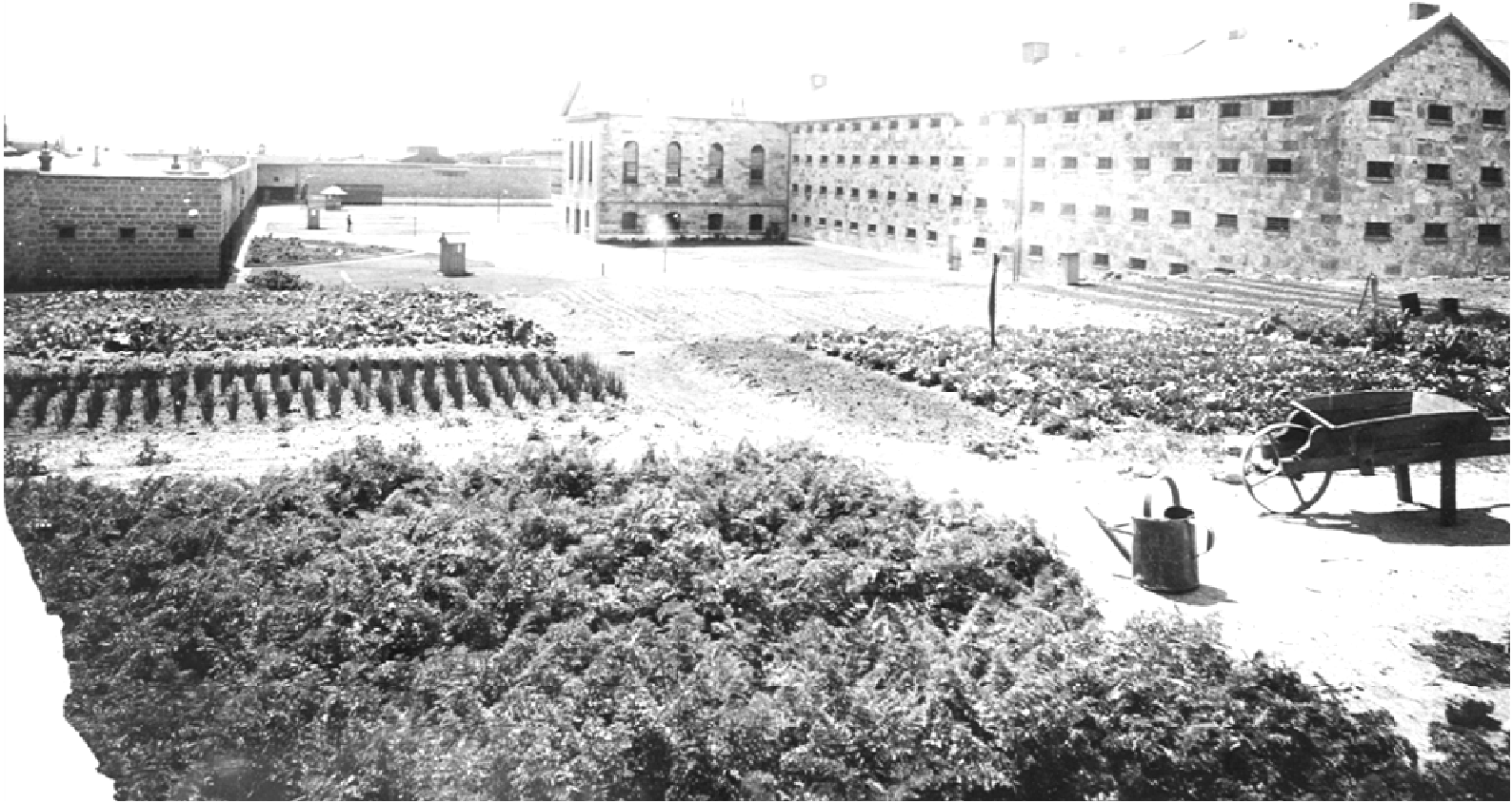
View of Main Cell Block from the South Knoll c1911 Fremantle Prison Collection
