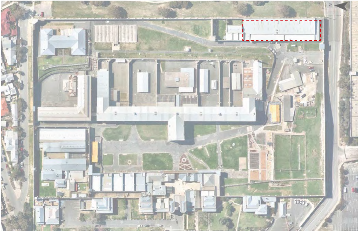
Figure 17. The East Workshops management zone indicated by the dashed red line.
