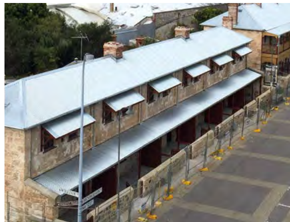
Above: Henderson Street Warders' Cottages.
