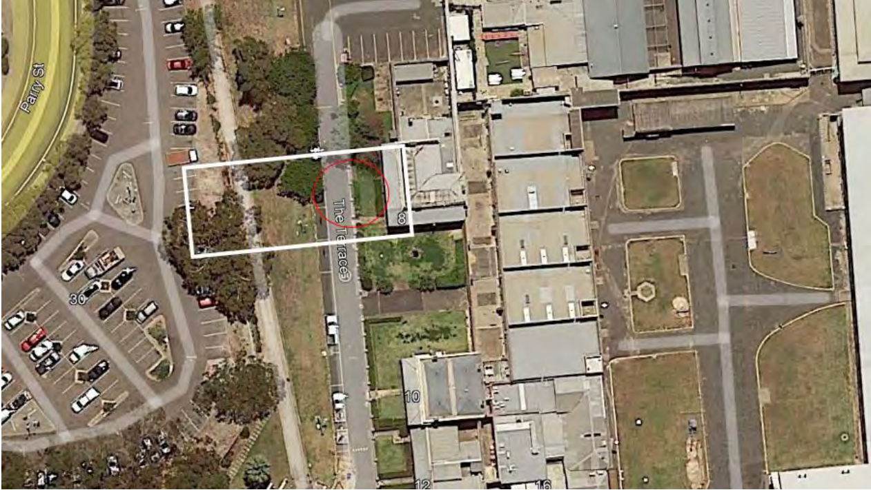
Figure 2. A general site map of the Fremantle Prison historical main sewer line area of interest outside the Fremantle Prison buildings (white rectangle and red circle) (image source: Golder).
