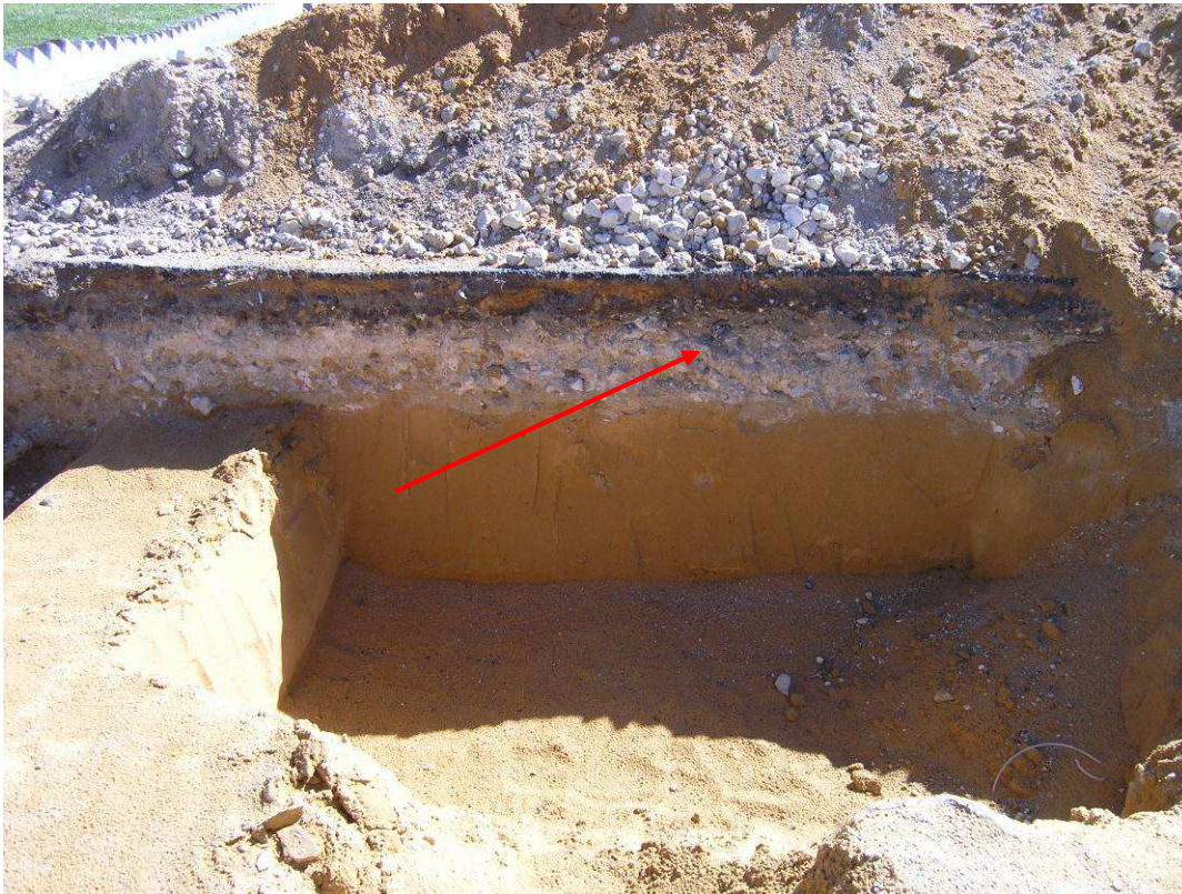
Plate 13. Area 5 (Metalled Road) – south facing section of trench. Crushed limestone layer (009) possibly original metalled road shown clearly in stratigraphy.
