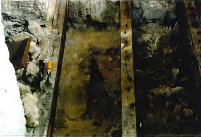
Plate 1. Cell drain during excavation
