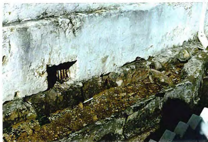
Plate 17. Drain outside Cell A20
