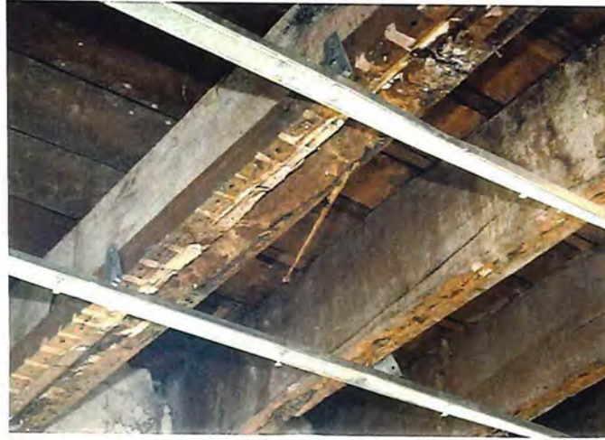
Plate 32. Repaired joist
