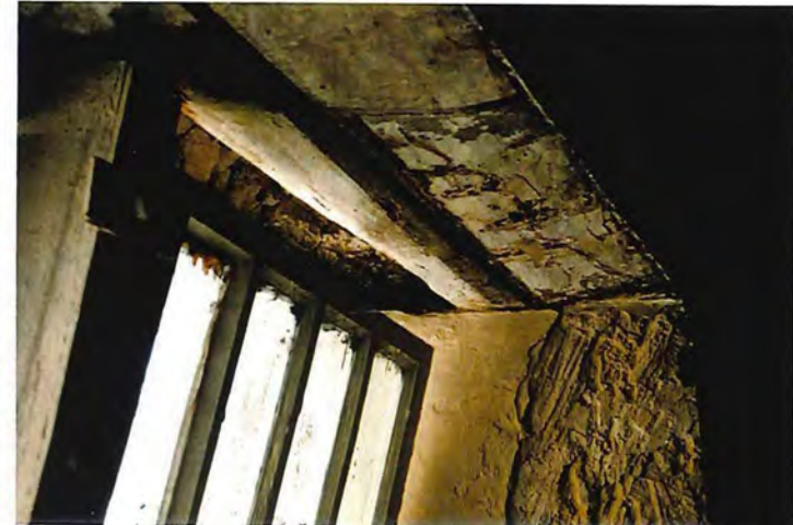
Plate 6. Original window lintel
