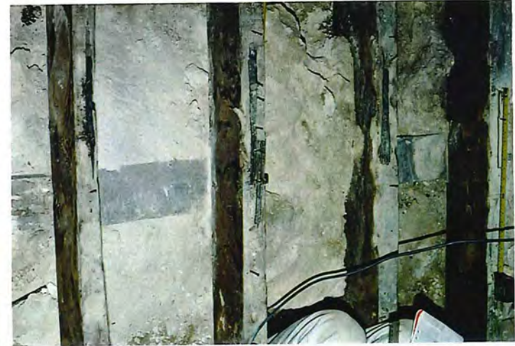
Plate 3. Bearer under joists
