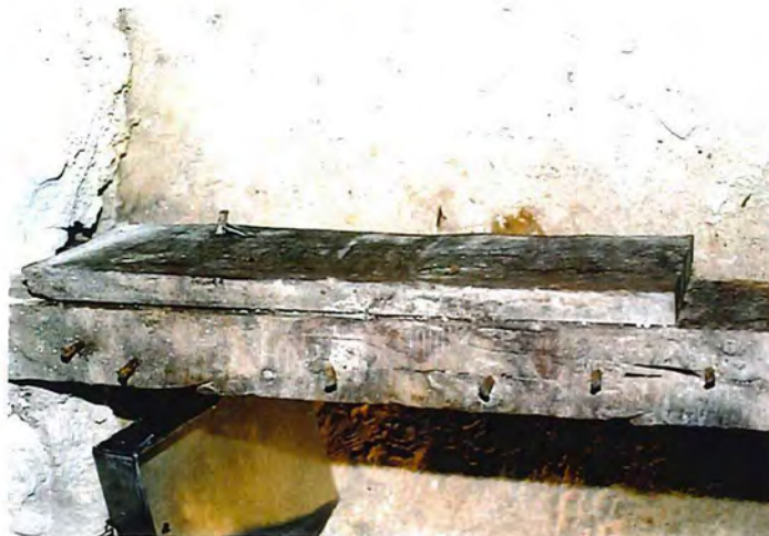
Plate 23. Joist repair
