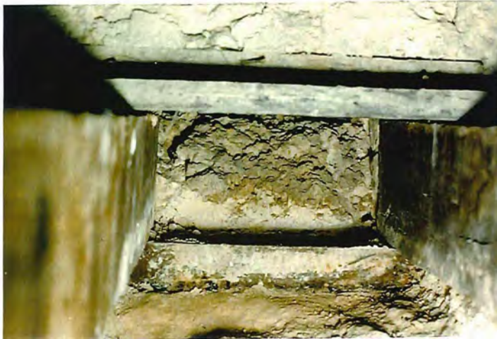
Plate 4. Inside under floor vent
