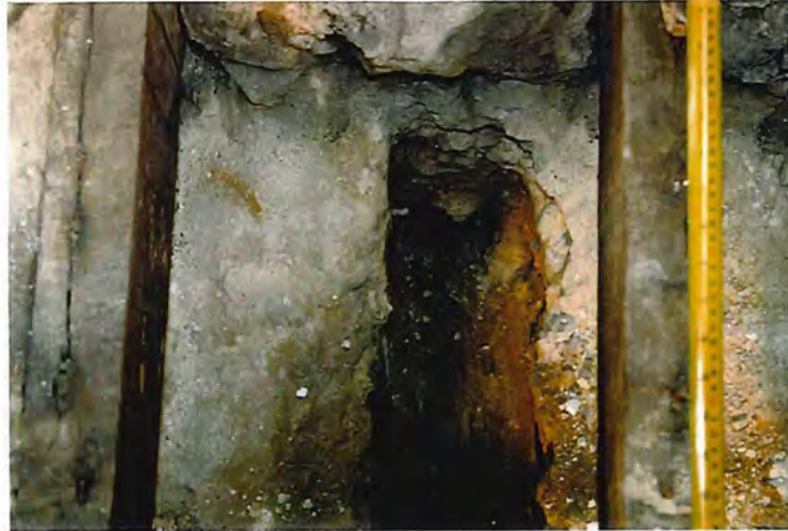
Plate 2. Cell drain fully excavated
