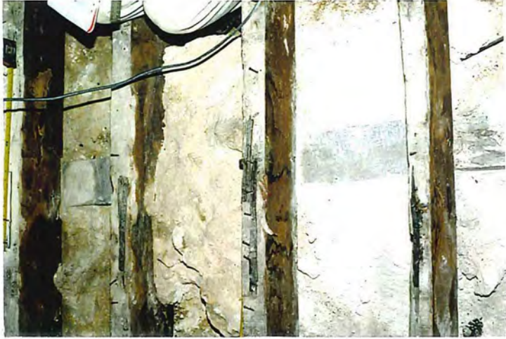
Plate 25. Battens over joists
