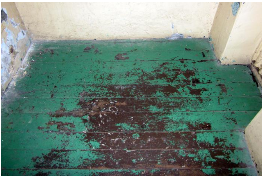
Cell A7 after floorboards replaced
