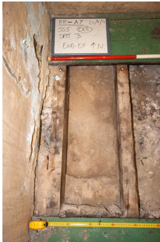
Joist space 5 end of excavation
