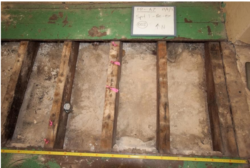
Joist spaces 1-3 prior to context 002 / Spit 1 excavated
