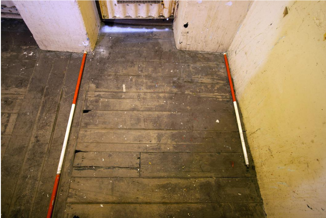
Cell F63 prior to floorboard removal
