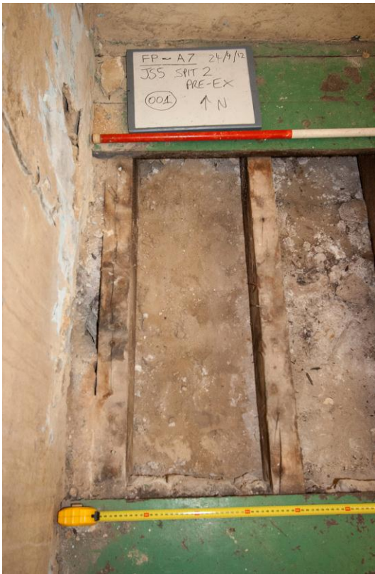
Joist space 5 prior to context 001 / Spit 2 excavated
