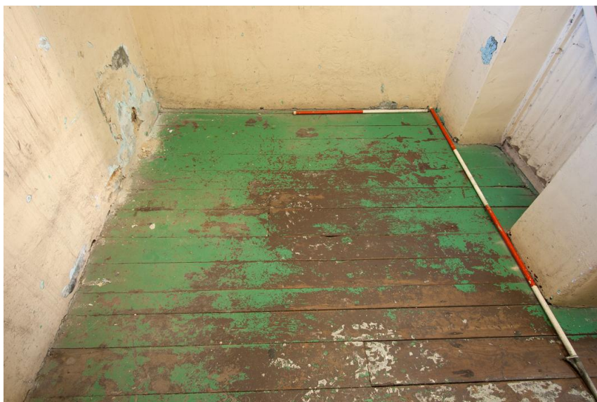
Cell A7 prior to floorboard removal
