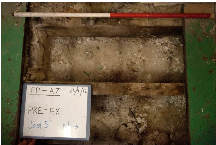
Joist space 5 prior to excavation
