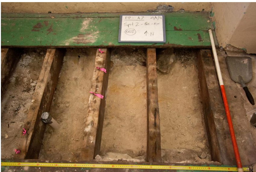
Joist spaces 1-3 prior to context 002 / Spit 2 excavated
