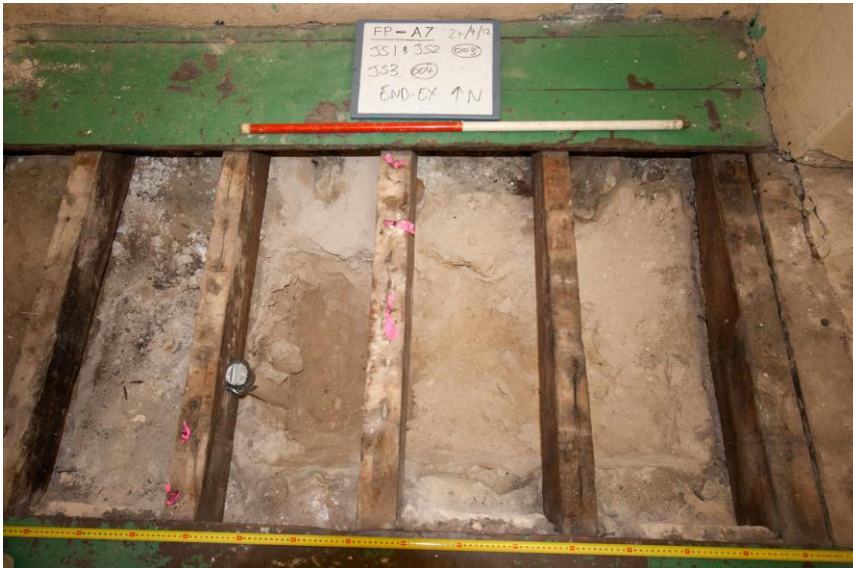
Joist spaces 1-3 end excavation
