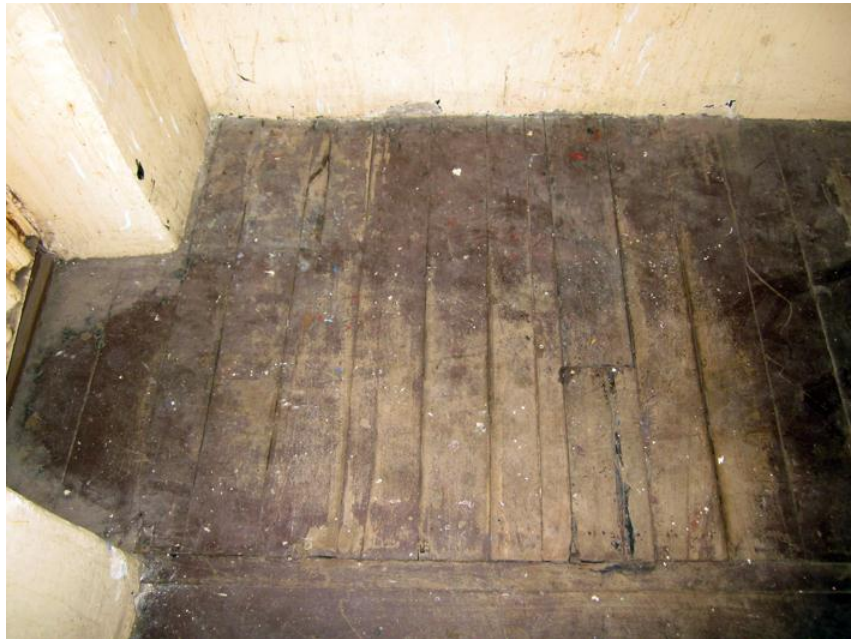
Cell F63 after floorboards replaced
