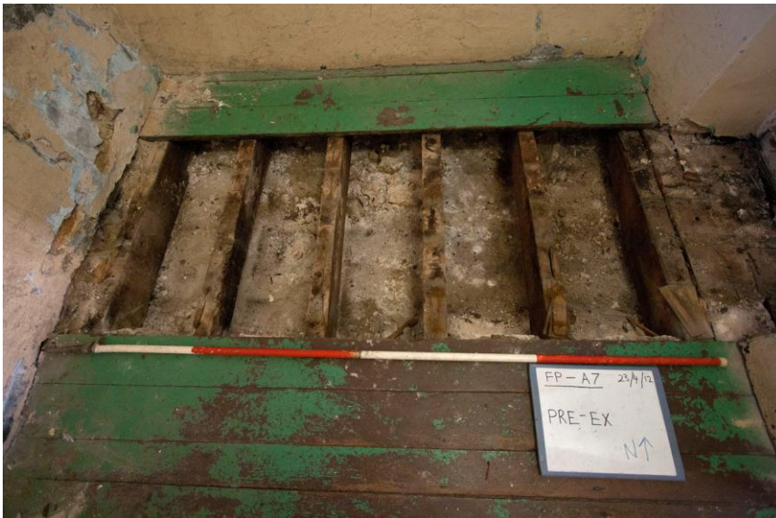
Cell A7 prior to excavation
