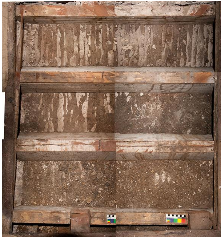
Photo mosaic of joist spaces 1 - 3 after embedded layer removed
