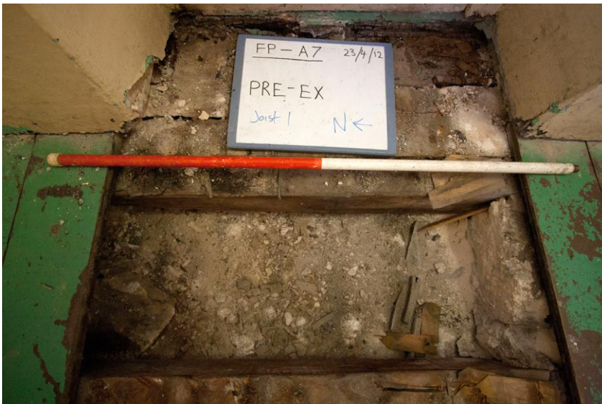
Joist space 1 prior to excavation
