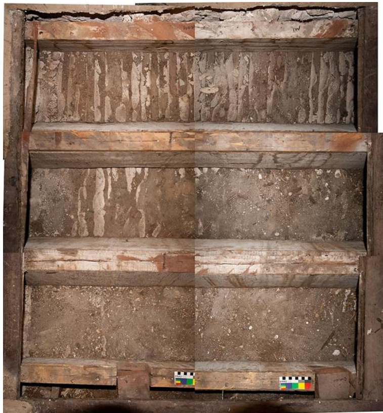
Photo mosaic of joist spaces 1 - 3 after 'spit 1' removed
