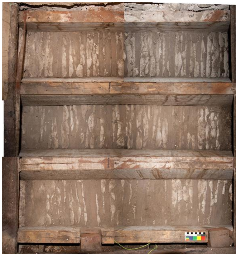
Photo mosaic of joist spaces 1 - 3 end of excavation
