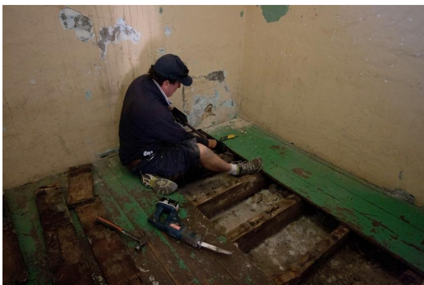
Removing floorboards
