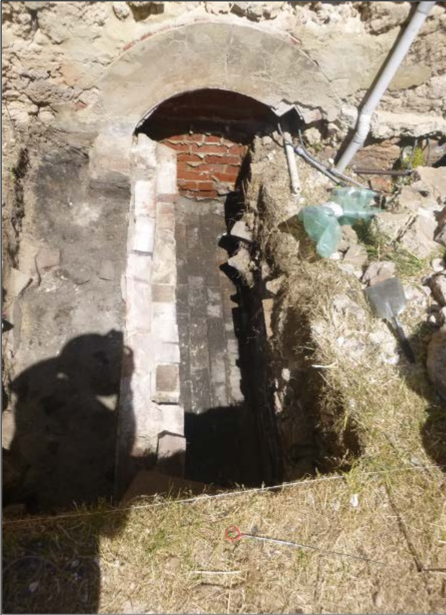
Figure 27: Brick floor of flue.
