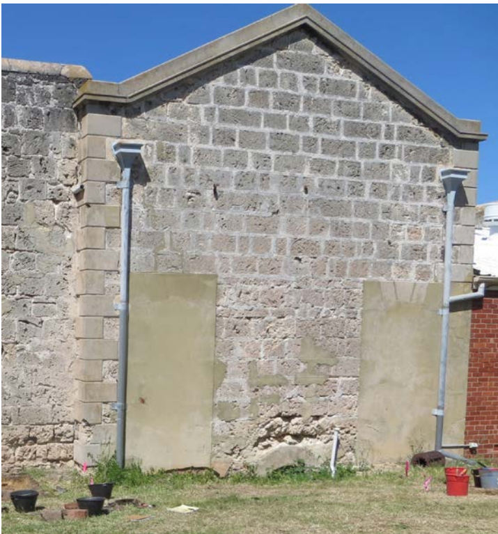
Figure 31: North wall of Engine House.
