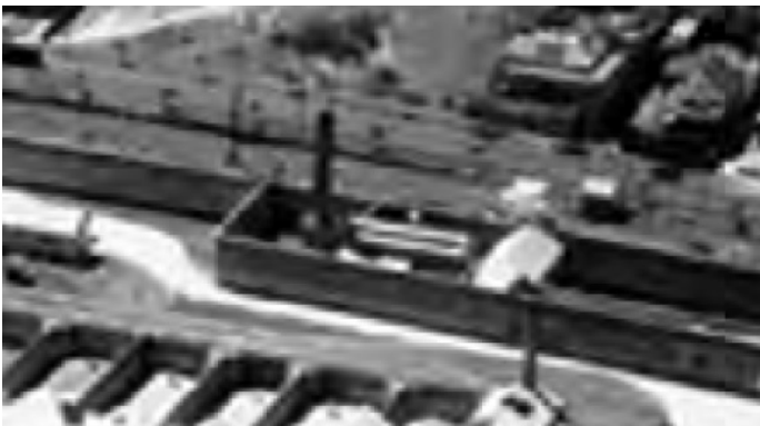
Figure 8: Detail from 1935 aerial photo showing Engine House and chimney.
