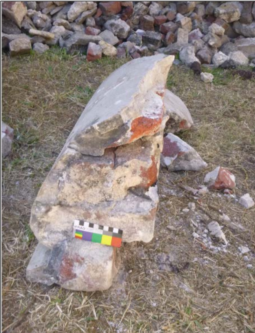
Figure 26: Domed brick and mortar structure: Roof of flue.
