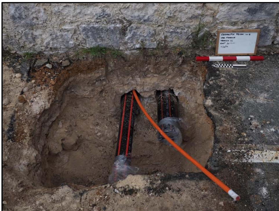
Plate 4: Service duct hole in western Perimeter Wall (Scale = 50cm)
