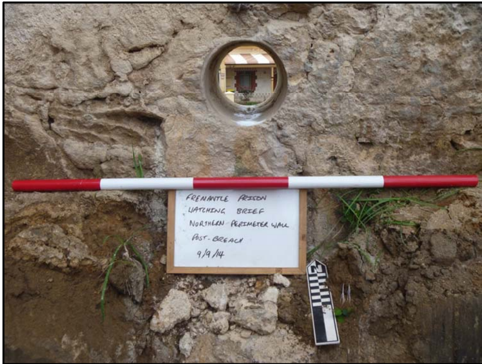
Plate 3: Service duct hole in northern Perimeter Wall (Scale = 1m)
