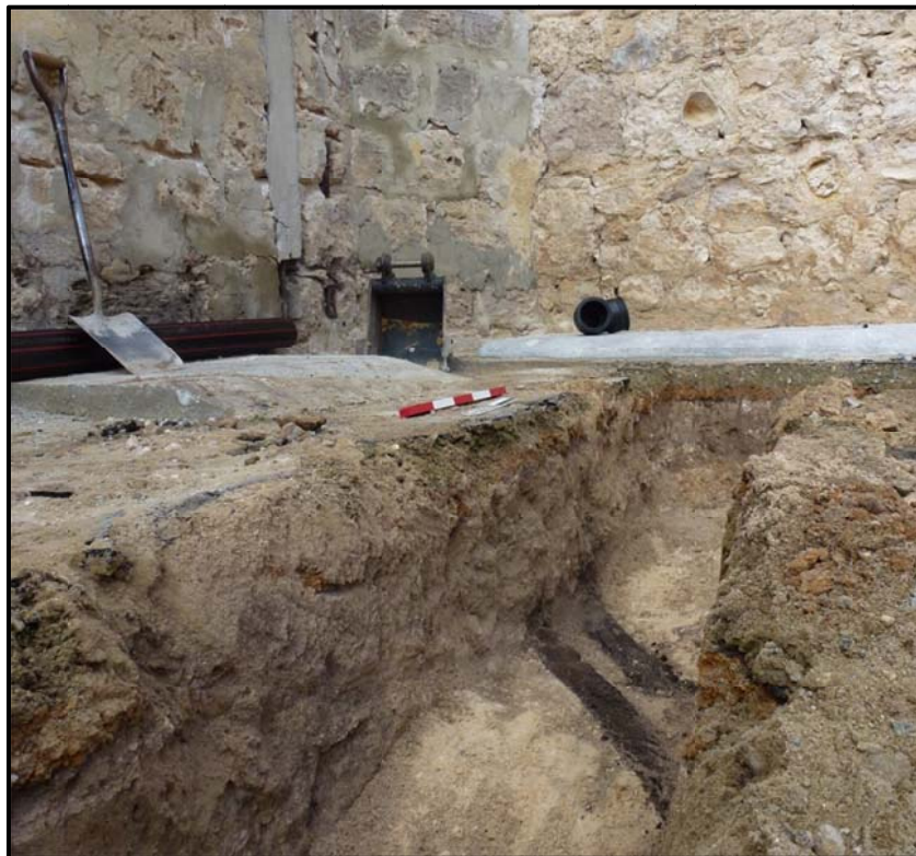
Plate 6: View of electrical feature C.118 in Trench ST6, looking southeast (Scale = 50 cm)
